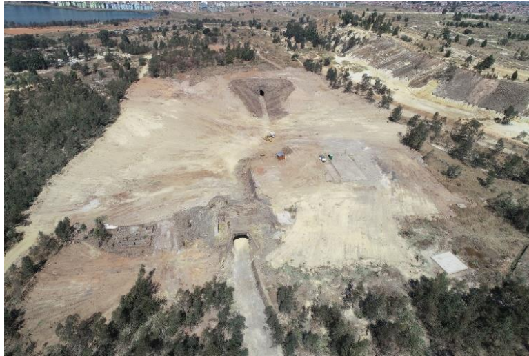
Image 1: Qala Shallows Site Preparation
