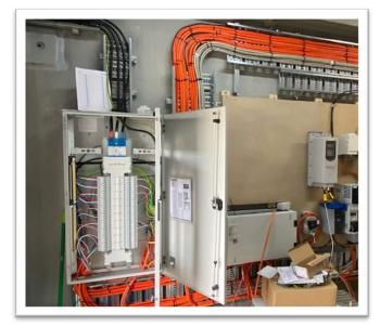
Figure 3: One of many connected power distributor boards
