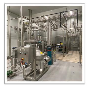
Figure 2: Completed and polished equipment and pipework
