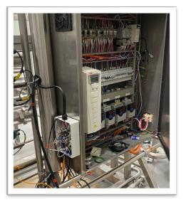
Figure 4: One of many PLC cabinets for equipment controls
