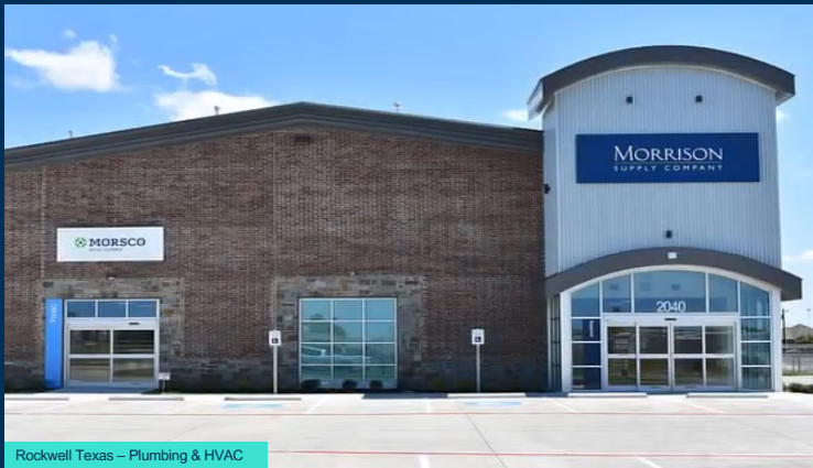
Rockwell Texas – Plumbing & HVAC
