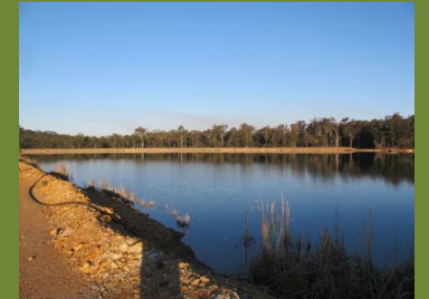
Mt Carrington Tailings Storage Facility
