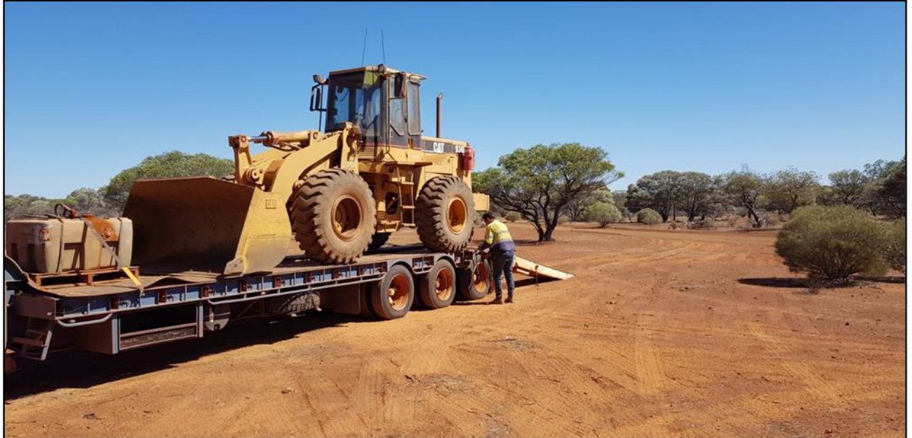
Golden Mile's Yarrabee Project, drill site preparation at Tank, November 2021
