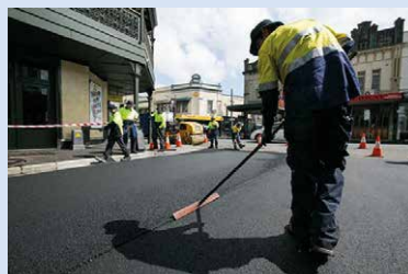
Figure 10: TonerPlas asphalt being laid in Australia.
