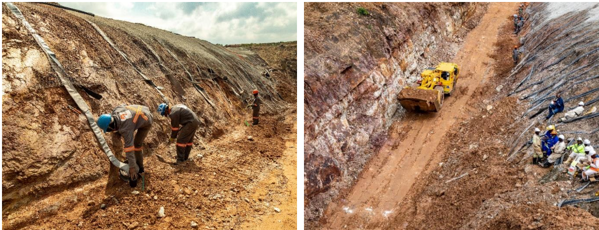
Image 3: Box cut rehabilitation
