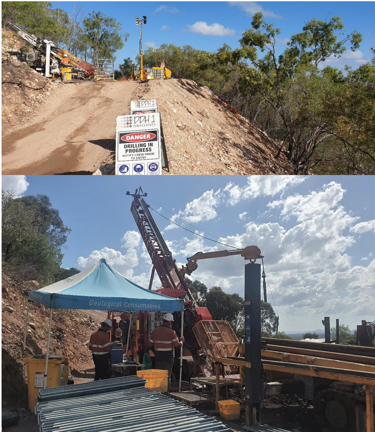
Figure 3: Drilling operations at BV7, December 2021.
