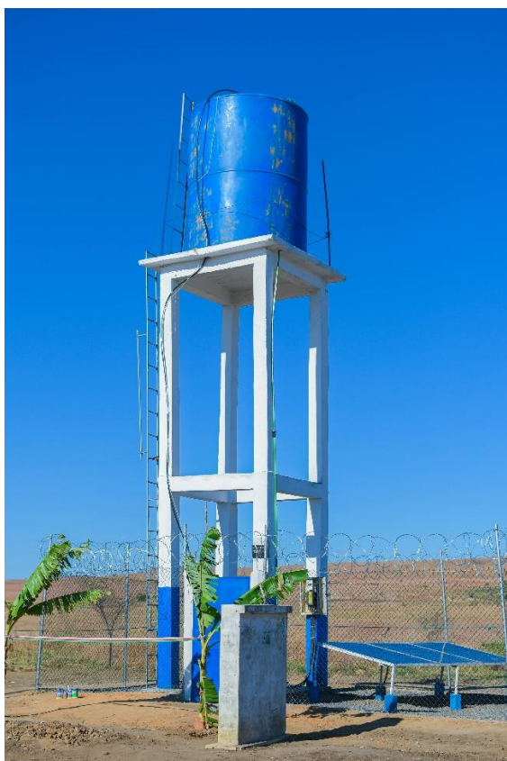
Water tower, water storage tank and solar panels for the water pump.
