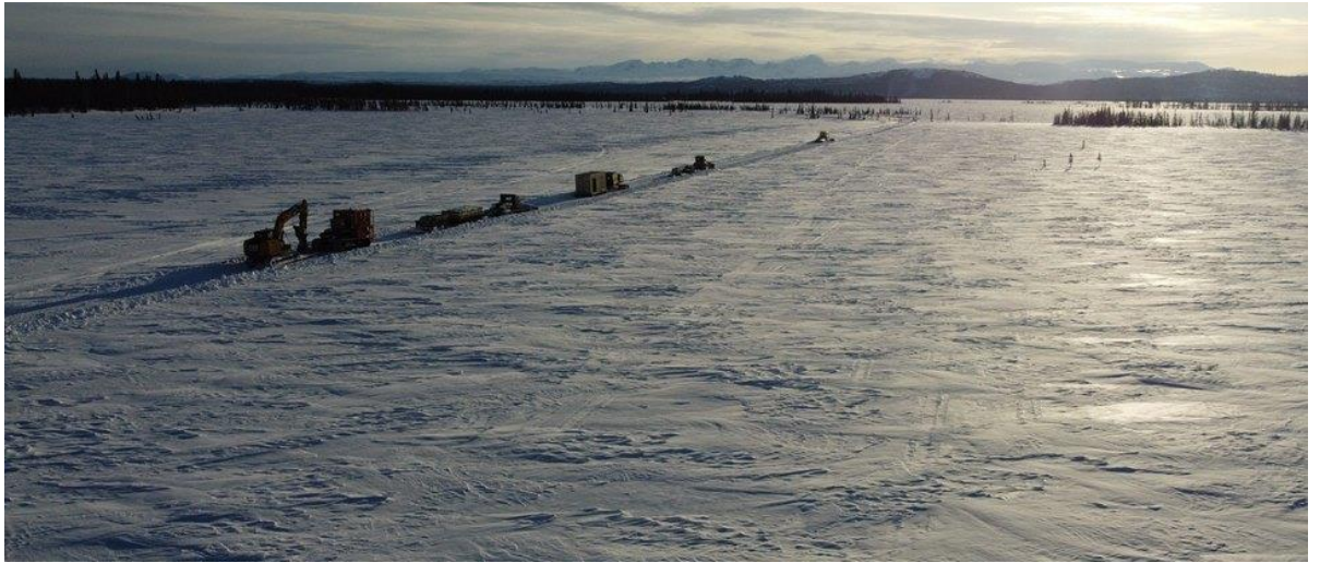
Figure 8a: Snow Road Operations Ongoing
