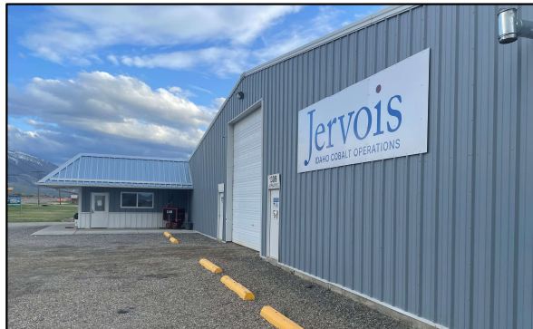
Salmon loadout facility
