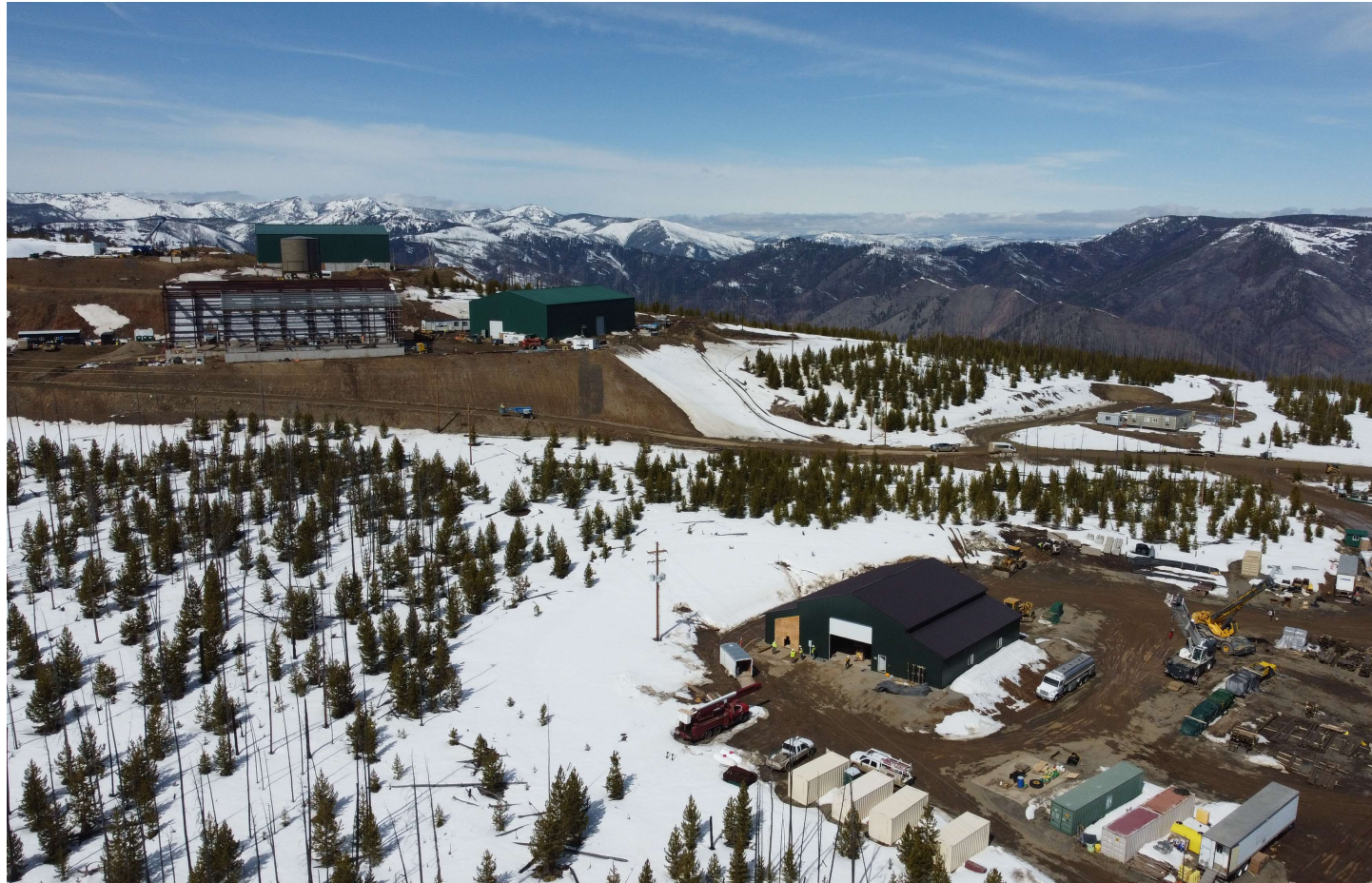
Surface Construction at ICO (March 2022)
