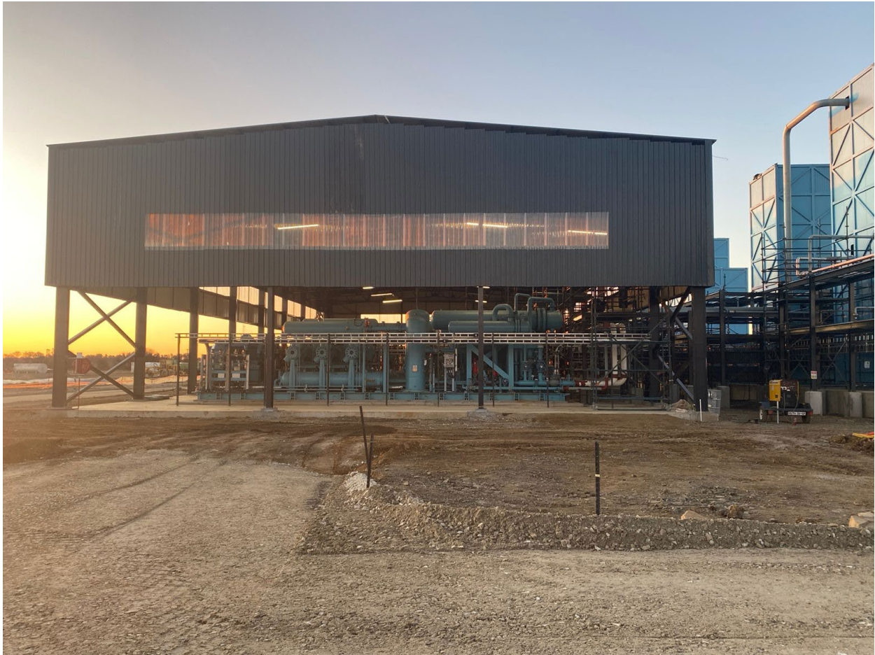
Images above of the main compressor building
