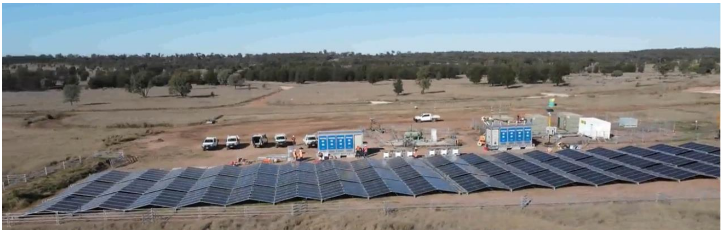
Figure 1: Site construction and acceptance testing in progress.
