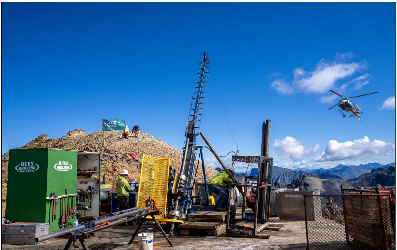
Figure 5. RPM South looking Northeast with drilling on Pad 6
