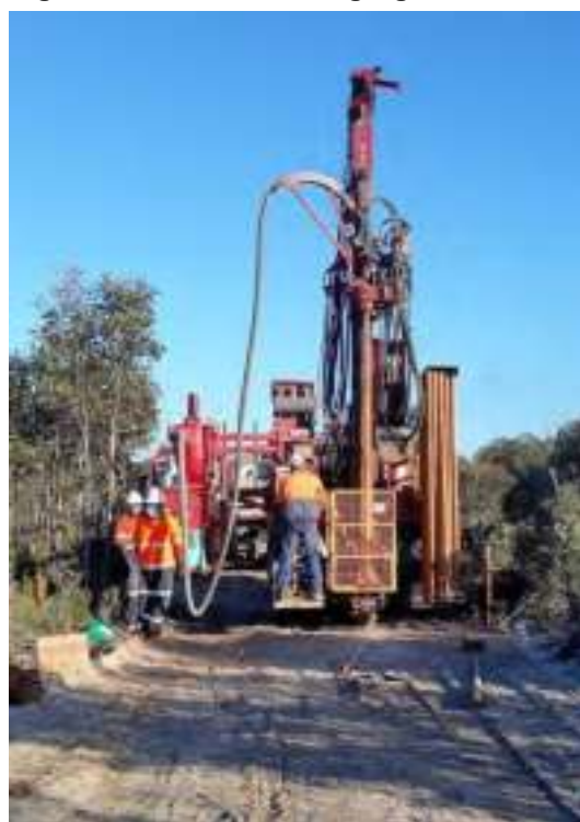
Figure 75 Air-core drilling rig
