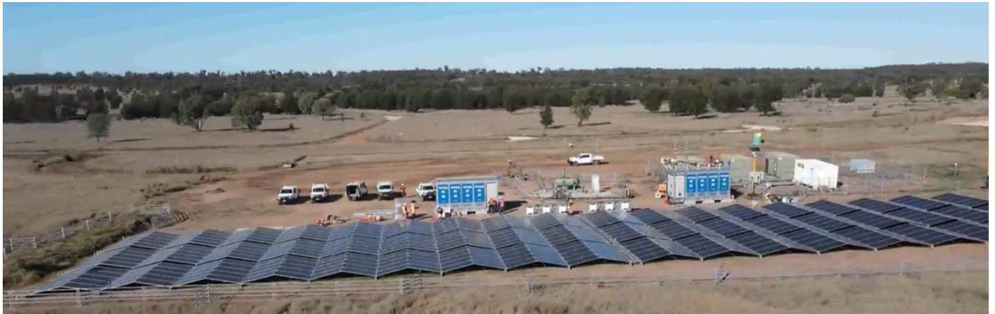
Figure 1: Site construction and acceptance testing in progress.
