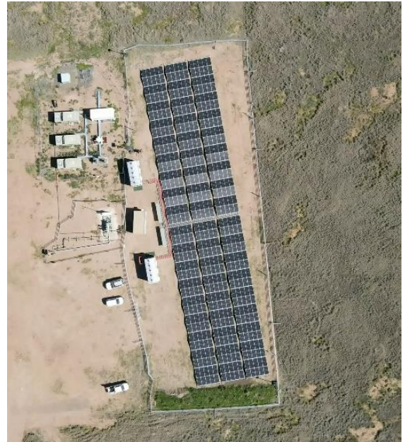
Figure 2: Aerial view of the Powerhouse site layout.
