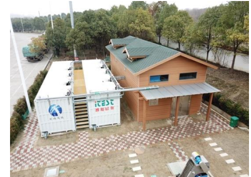
Highway rest stop Aspiral L4 plant, Xiaogian, Hubei province
