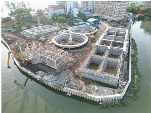
World’s largest MABR plant in construction in Sihanoukville, Cambodia
