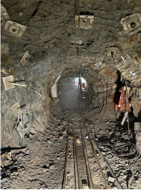
Figure 2 – Ore haulage level – rise miner in background.
