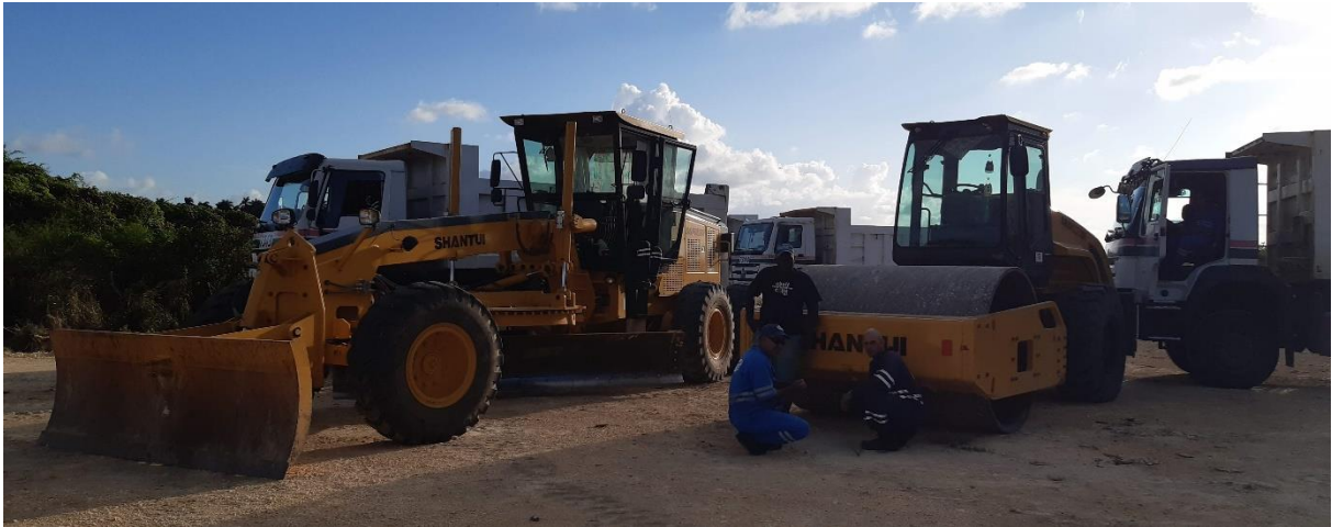
Figure 2 - Civil contractors arriving at the Alameda well pad to commence work
