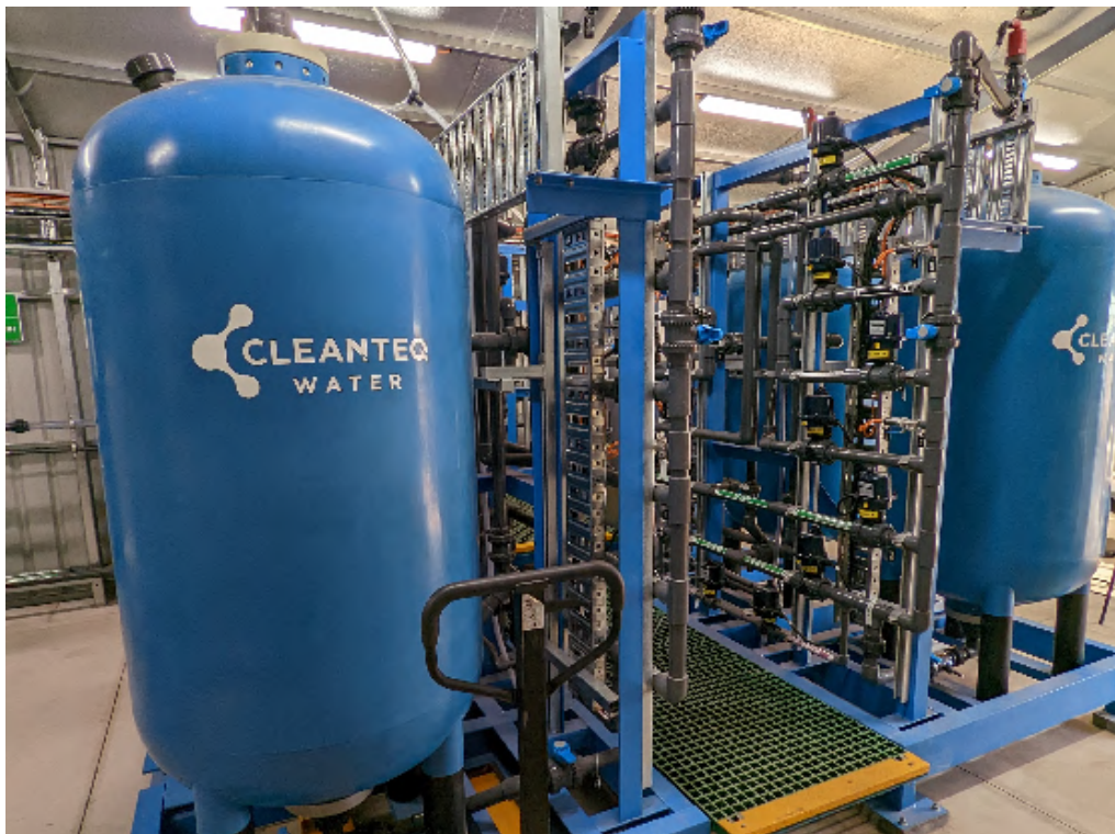
Clean TeQ Water's ion exchange water treatment plant (Laramba)
