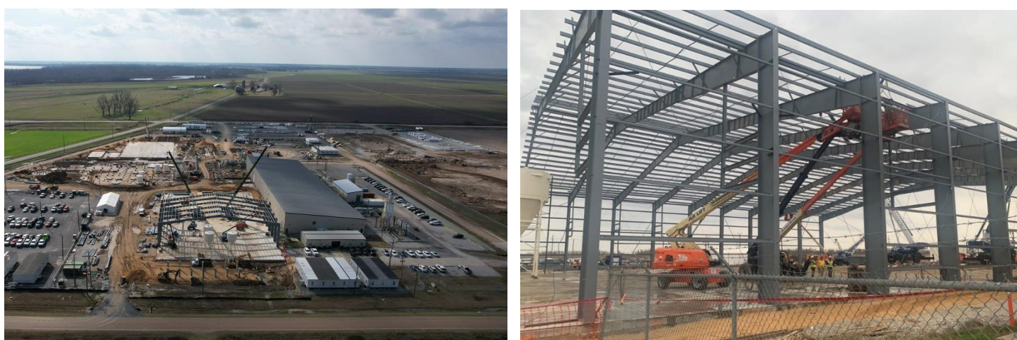
Figure 2: Construction of 11.25ktpa AAM Vidalia facility.
