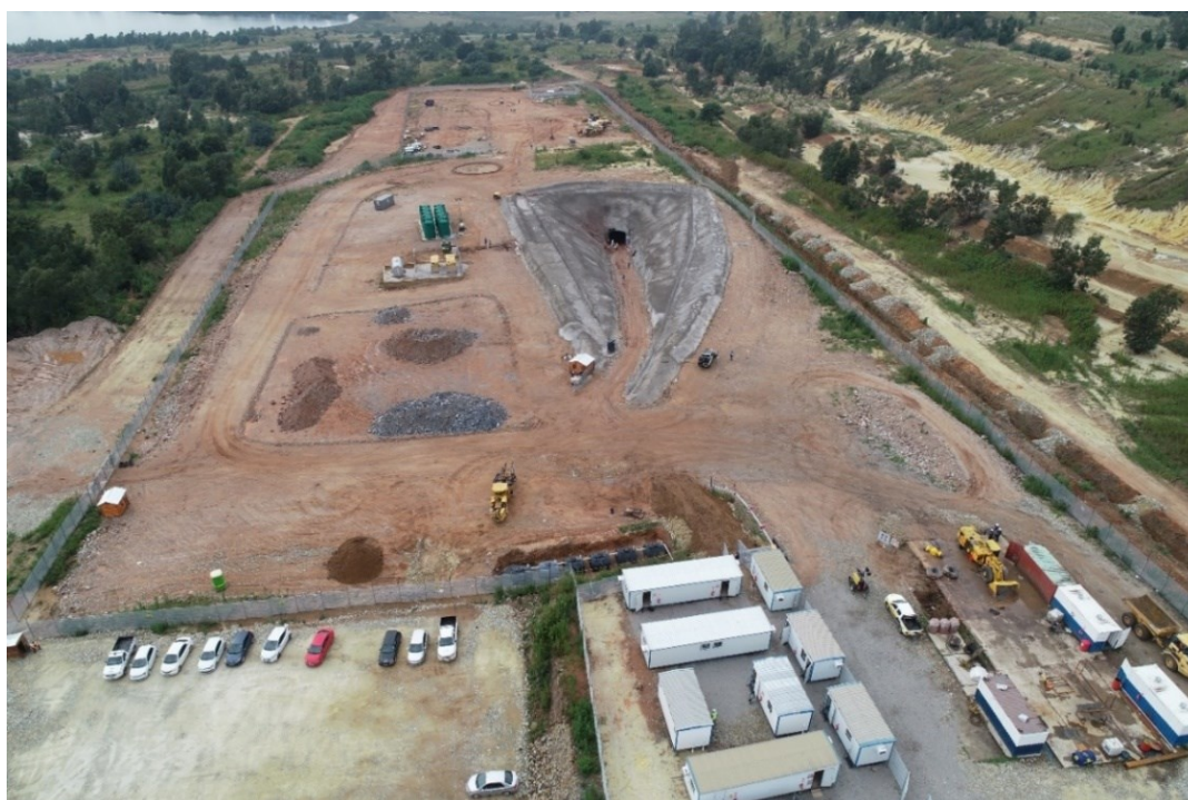
IMAGE 1: PHASE 1 QALA SHALLOWS INFRASTRUCTURE
