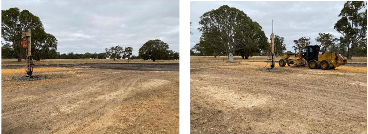
Figure 8: Killanoola site works, January 2023
