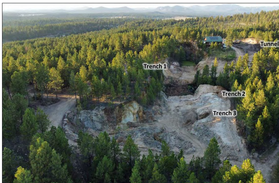
Figure 5 - Aerial view showing the three trenches cutting the base of the historic mining operation at Longview.
