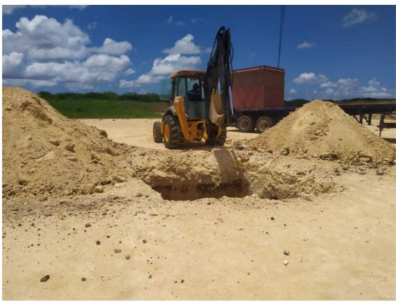
Figure 2 - Construction of the cellar prior to the installation of the conductor
