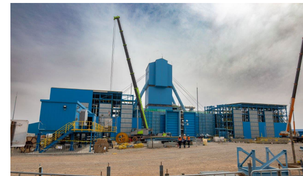
Shaft 3 mine air heaters
