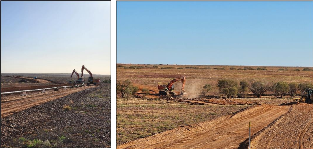
Figures 4-5: Yarrow 3 Pipeline under construction June 2023. Photos show pipeline being buried.
