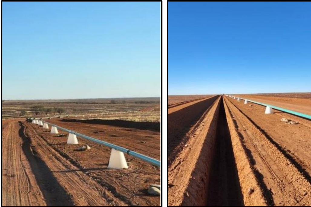
Figures 2-3: Yarrow 3 Pipeline under construction May 2023
