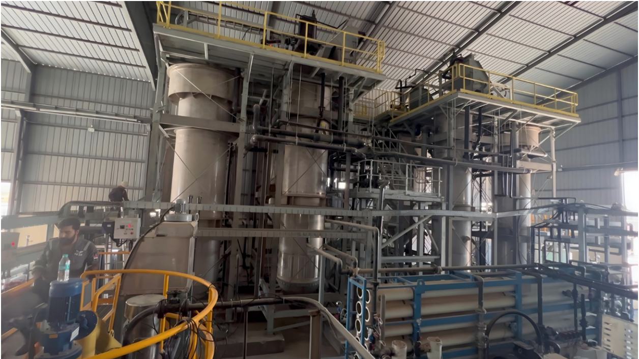
Commissioning of the NESR HIROX® project underway
