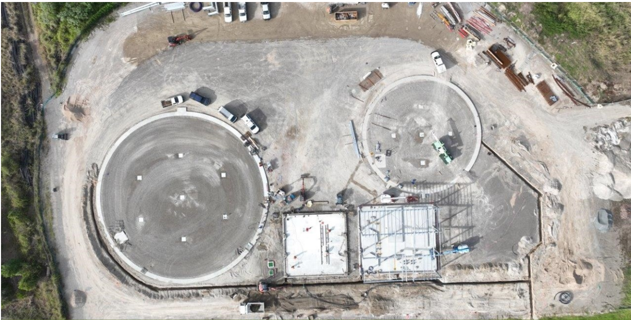
Finished concrete slab and shed nearing completion on site in Townsville
