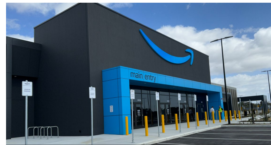
Amazon, Jandakot Airport industrial precinct, Perth WA
