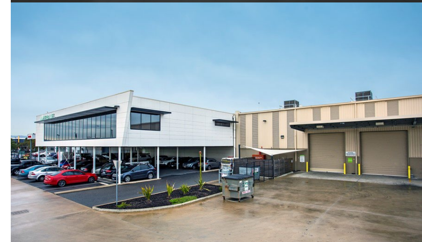
20-22 Butler Boulevard, Adelaide Airport SA
