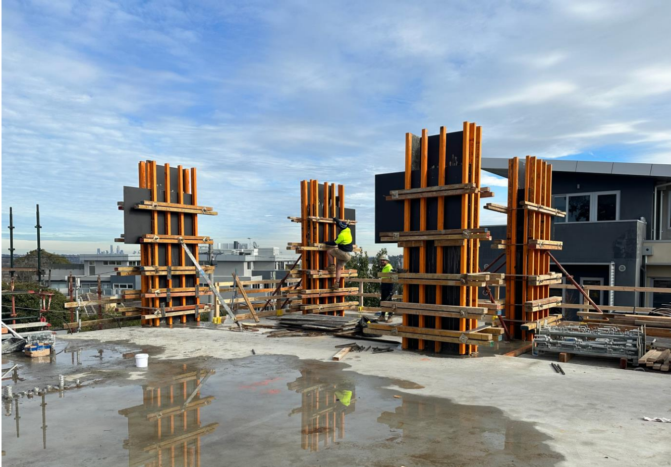
Genius Childcare - under construction, Templestowe Lower, Vic
