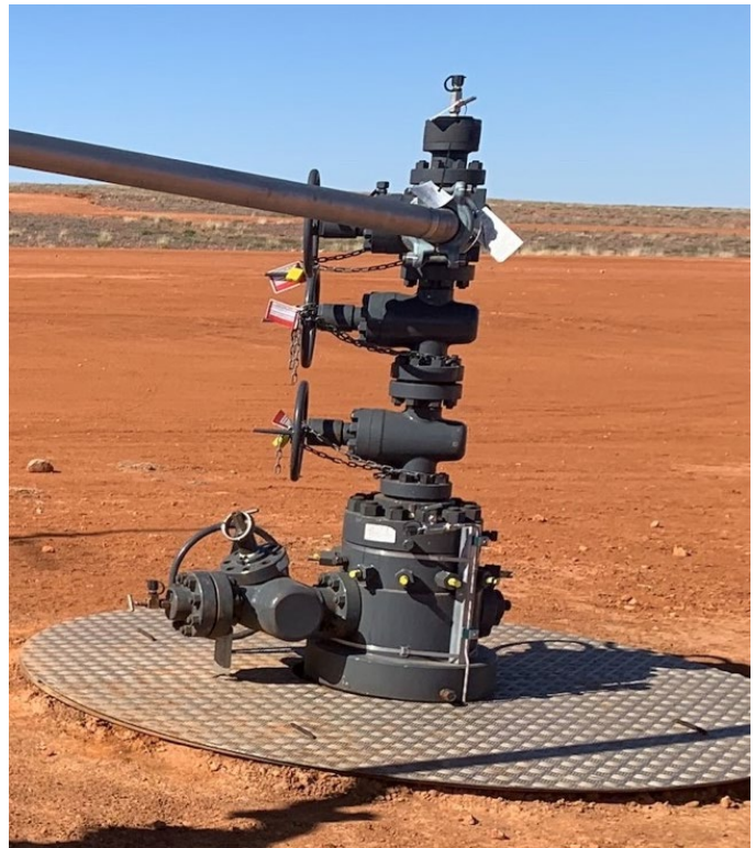
Figure 1: Wellhead at Yarrow 3 (Courtesy of Santos)
