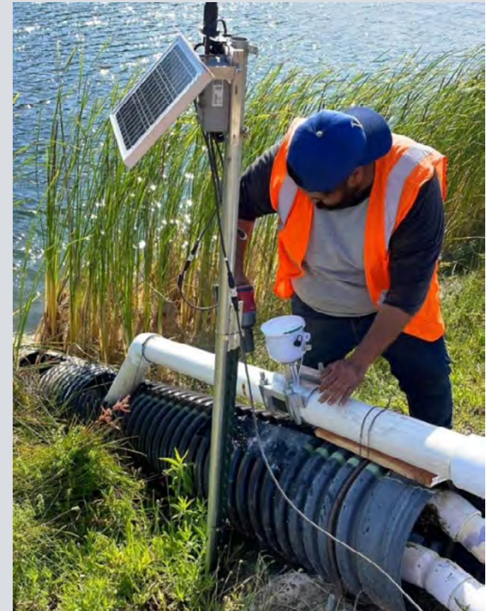
Installing a new flowmeter and data logger telemetry unit with a solar panel used for power at our Beaulieu Vineyard 2 in the US
