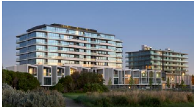
Waterline Place Williamstown, Victoria 184 remaining IH & APT lots
