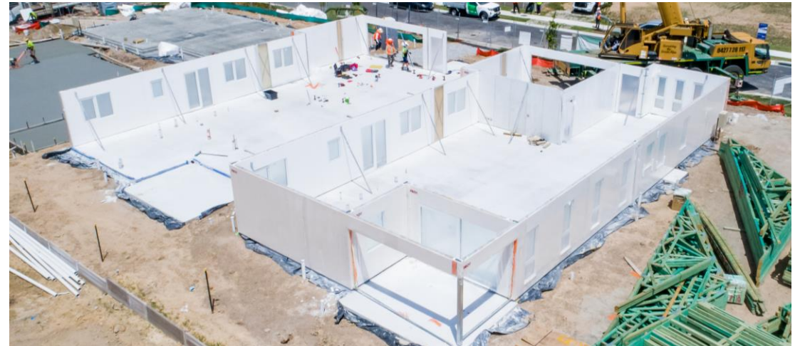
Construction of home with Pro9 walling system
