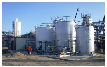
Figure 4: 11.25ktpa AAM Vidalia facility purification area (left); water and neutralisation discharge tanks (right).
