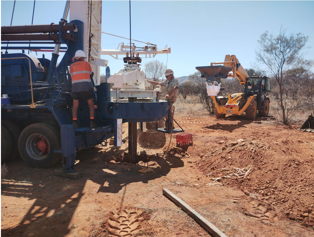
Above: Drilling with bucket drill, telehandler awaits discharge of bucket
