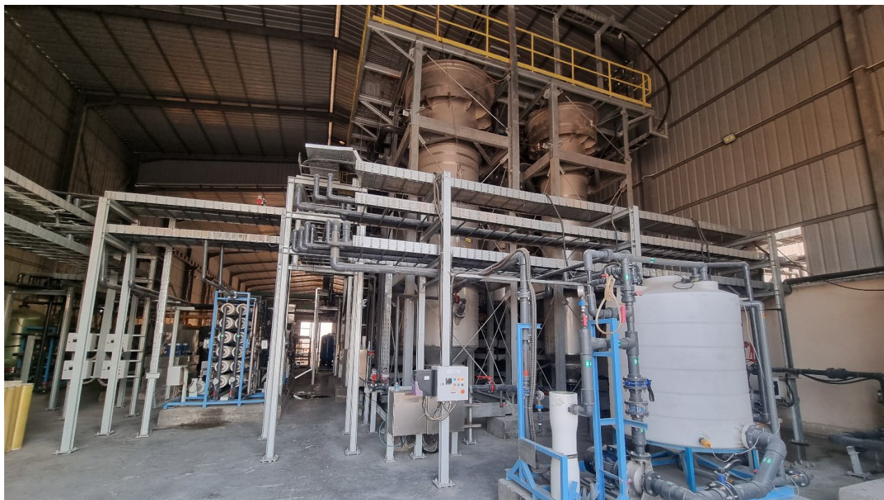
Photo of the HIROX® plant during commissioning in the Middle East
