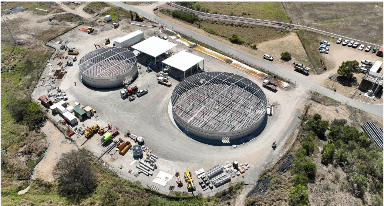
Photo of installation progress at Townsville
