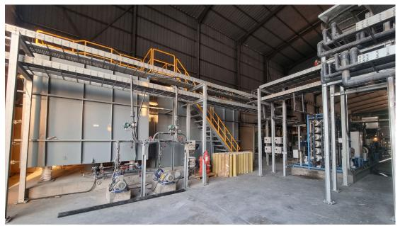
Photo of the brine recovery circuit of the HIROX<sup>®</sup> plant
