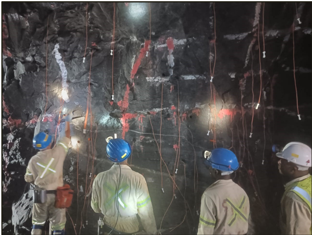
Photo 3: +105 Level face charging.
