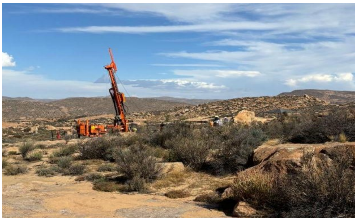
Photo: Drilling in progress at OCP.
