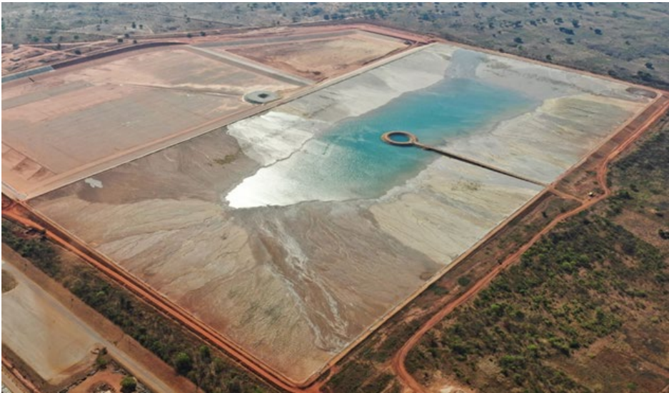
Tailings storage facility (cells 1 & 2)
