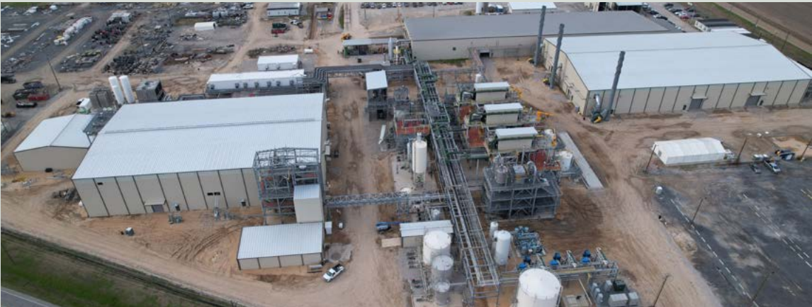
◀ Vidalia AAM facility
