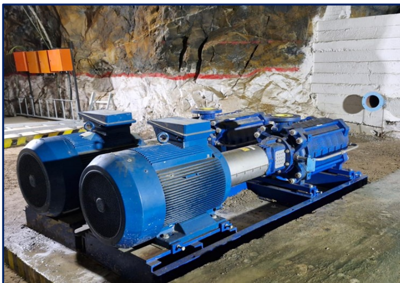
Photo 3: Underground 178m Level Multi-Stage Pumps.
