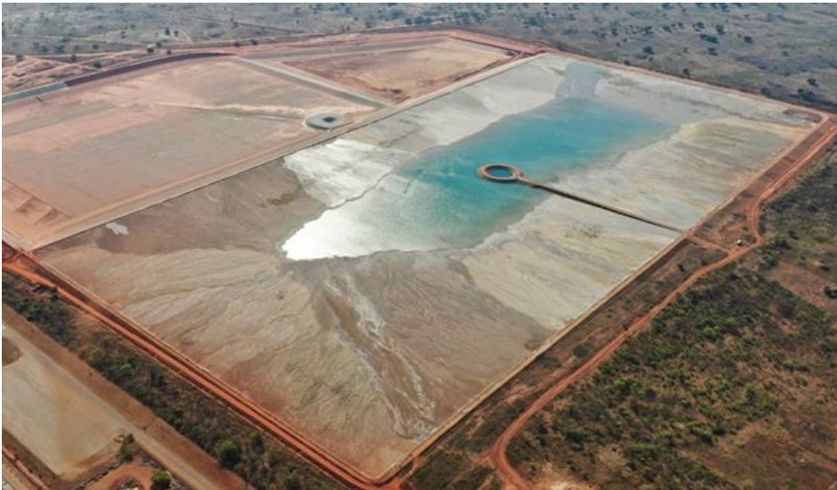
Tailings storage facility (cells 1 & 2)
