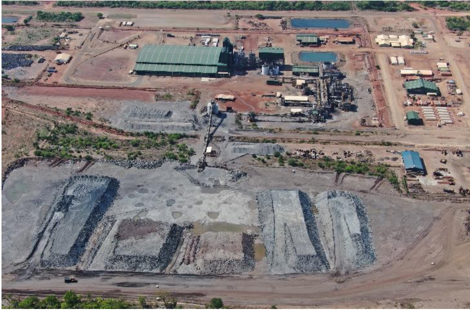
Process plant, product warehouse and ROM stockpiles
