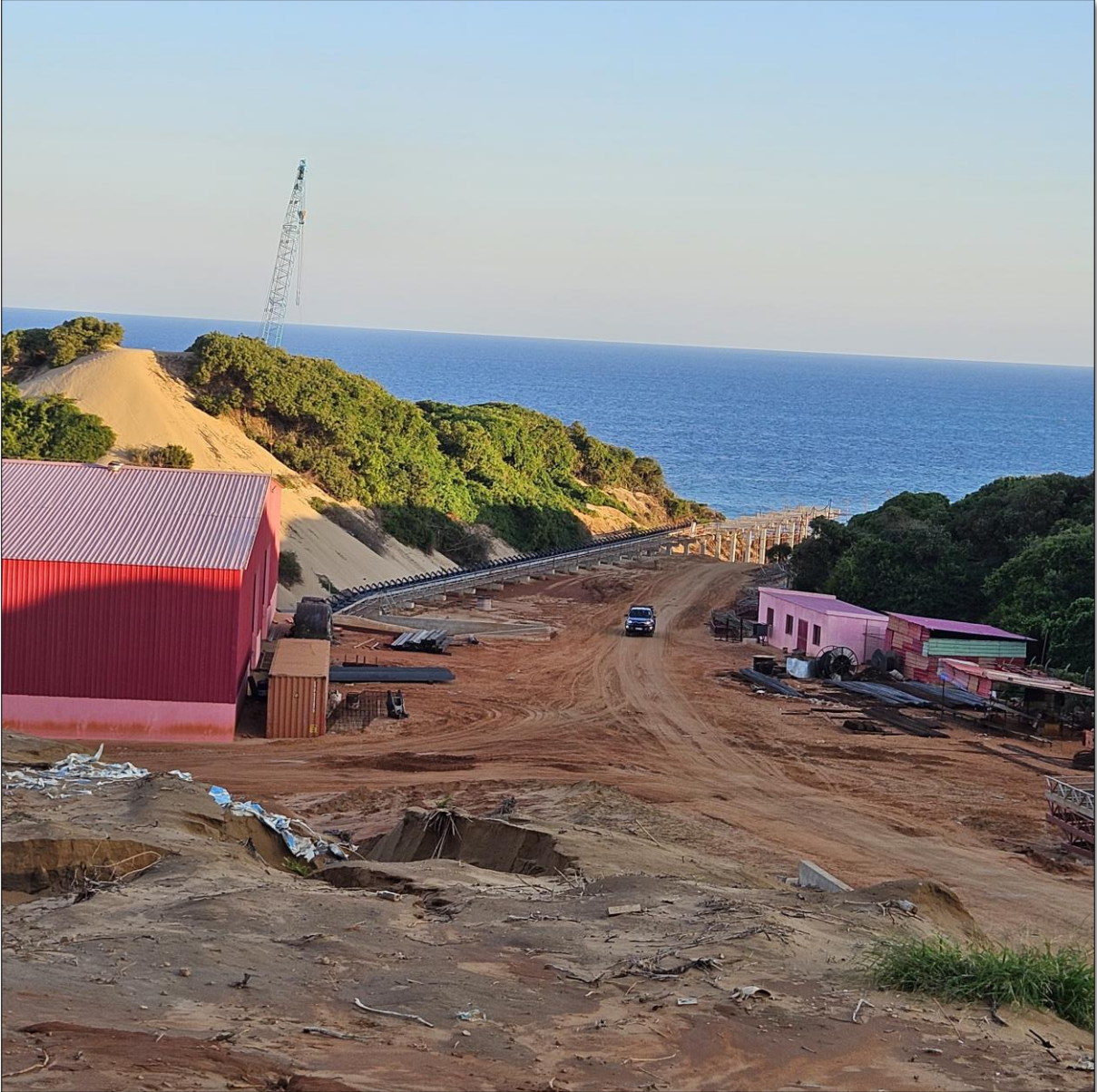
Figure 2: New HMS loading jetty under construction at Chongoene.
