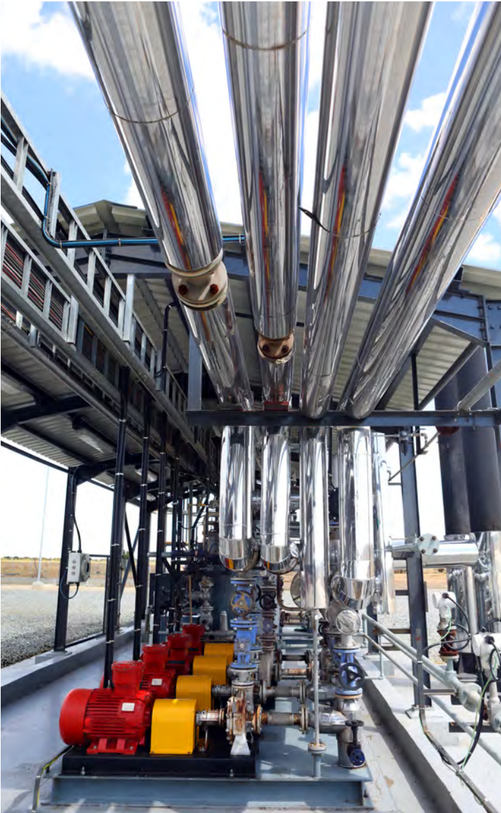
Conduction oil pumps.
