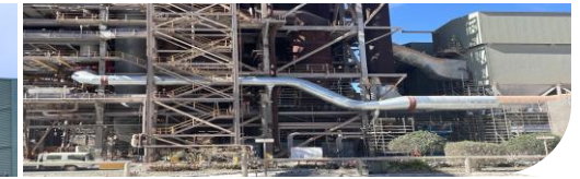
Hydrogen calcination pilot Construction is underway at Yarwun for this world first technology
