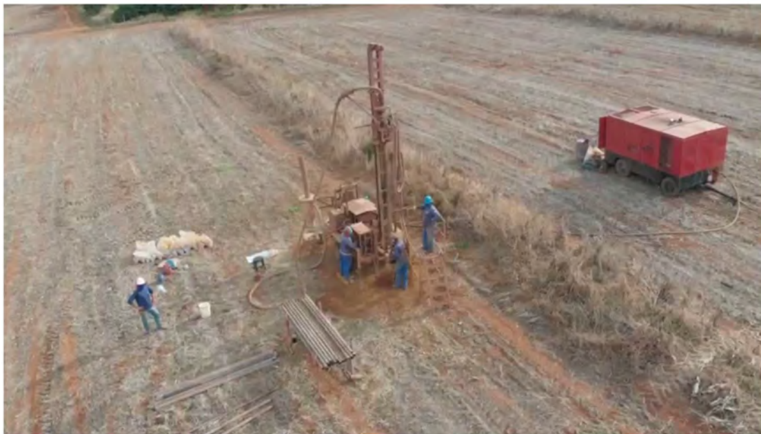
Figure 4: RC Drilling in action supported by drilling crew (Drone footage)
