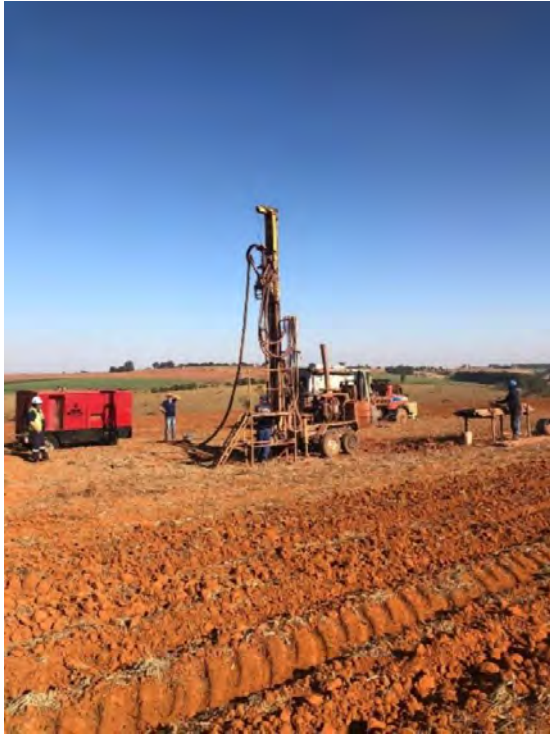
Figure 6: RC drilling in operation in CODA North
