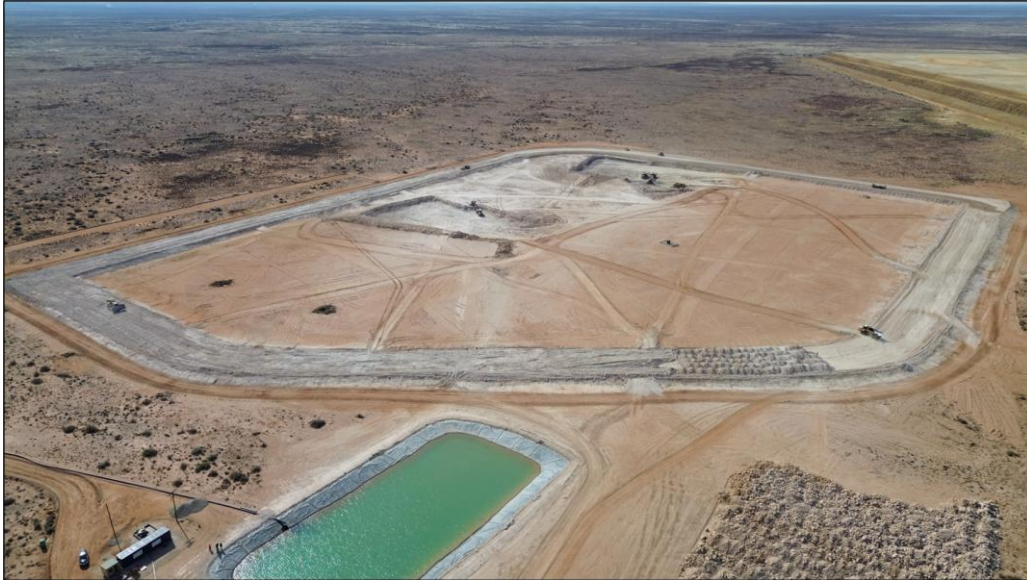
Photo 2: 13ha Water Storage Dam on 65ha TSF footprint.
