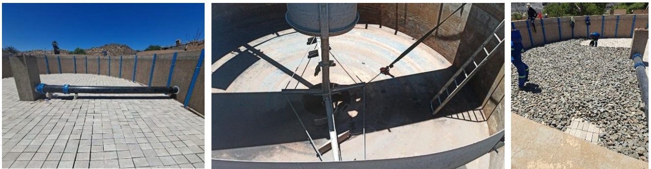
Photo 3: Images showing refurbishing works to the Biofilters and Clarigesters in progress.
